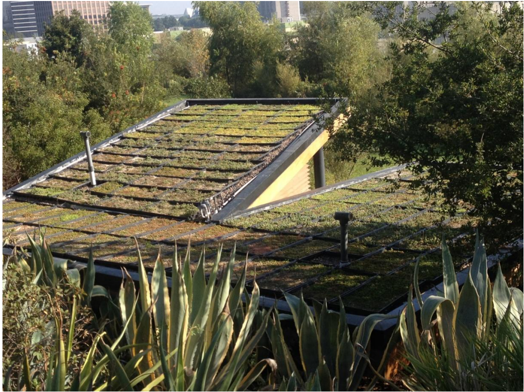
Image 1.6: Green Roof of Bathroom and Native Landscaping. Photo by Allie Rigby, 2013.
